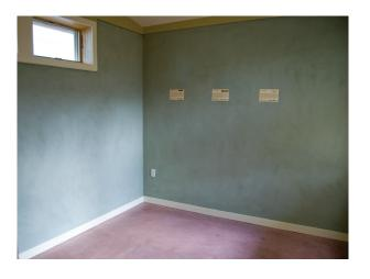
reconnect to this history. Composed of 100% natural earth plasters, it provides a durable and unique finish that has been applied over a mud-clay substrate containing soil which was excavated from the West Hills of Portland only hours before its application.
