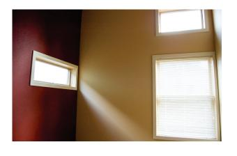
frames and double pane Low E II insulating glass with argon gas. More durable than vinyl with a lower thermal expansion rate than aluminum or wood, this assembly provides a tight seal with an overall u-value of .29, compared with an average u-value of .48 that is found in typical new residential window systems.
